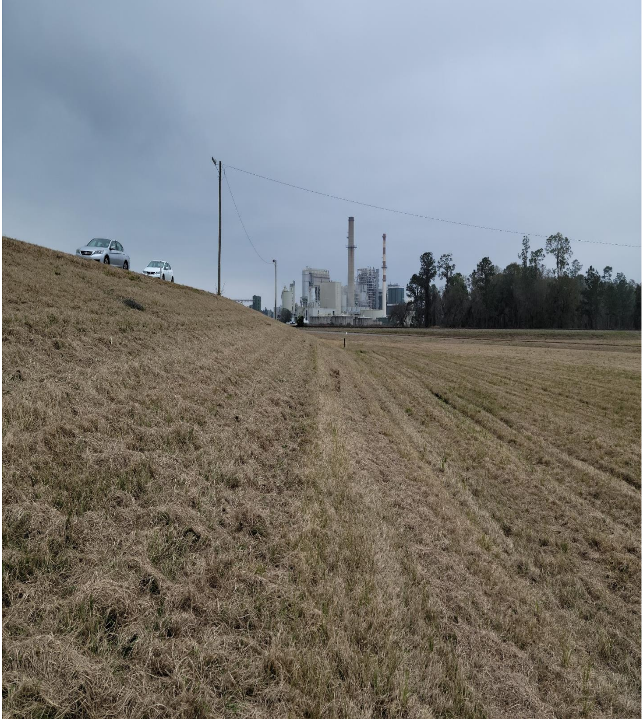
Figure 3. Trimmed grass on the southern slope of the surface impoundment system; 01/27/2021.
