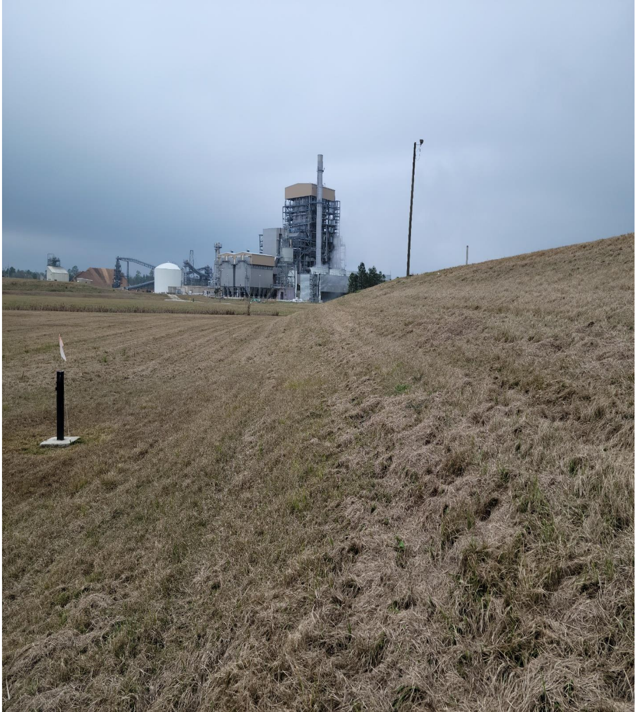
Figure 2. Trimmed grass on the southern slope of the surface impoundment system; 01/27/2021.
